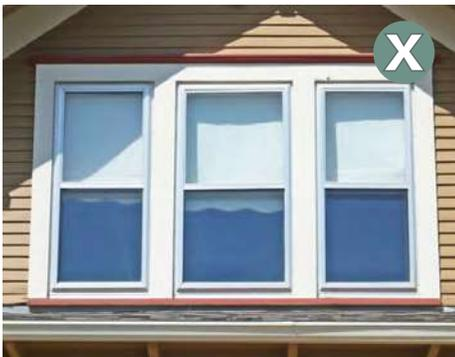
Unfinished metal windows such as these alter the character of window openings, and should not be used in highly visible locations.
