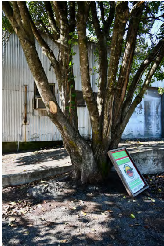
Low trunk structure of tree #1.
