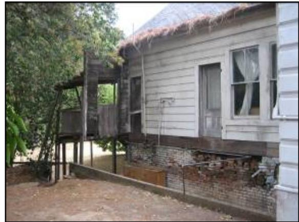
*Example of deteriorated foundation and siding*
