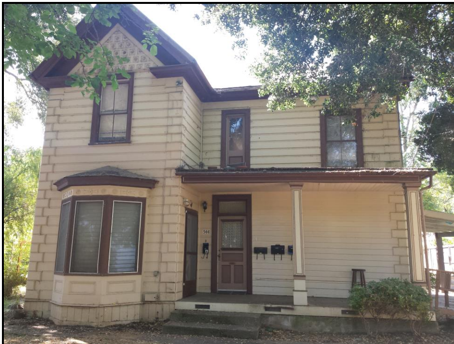
N elevation of residence, showing door added to the east of original door when house was converted to 3 flats in the 1920s, photo view toward S, 12/2017.
