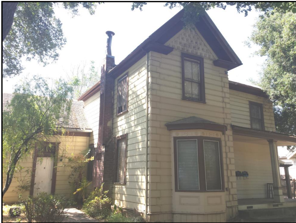
N elevation of medical office addition and E and N elevation of residence, photo view toward SW, 12/2017.
