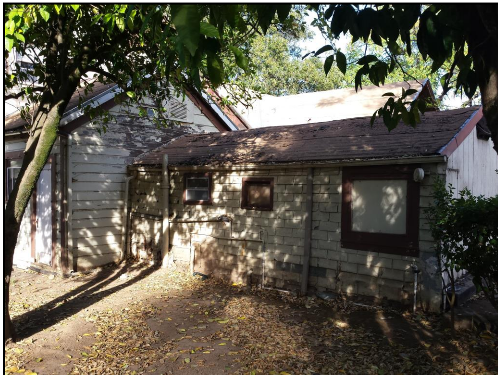
Close up of W and S elevations of additions on W side of residence, photo view toward NE, 12/2017.
