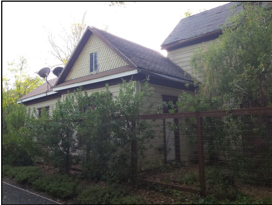
E and N elevations of 1890s doctor office addition with a later cross-gabled S addition that matched the previous quality of windows and siding, but not fish scale shingles; photo view toward SW, 12/2017
