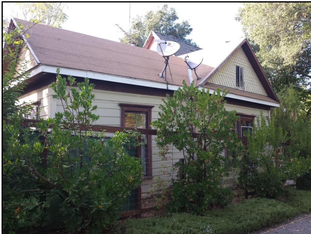
S and E elevations of the cross-gabled later addition to the one-room doctor office, photo view toward NW
