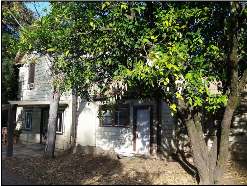
W elevation of residence and additions, photo view toward NE, 12/2017
