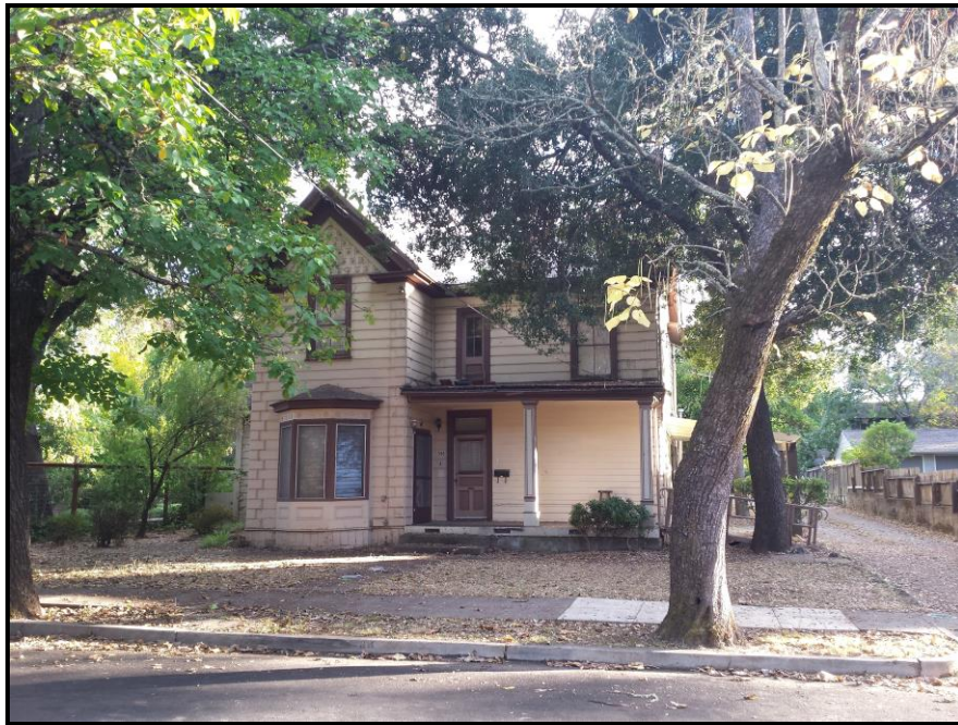
North Elevation, December 2017
