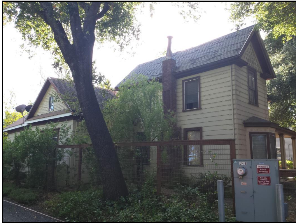
E elevation of residence and 1890s doctor's office addition, photo view toward SW, 12/2017
