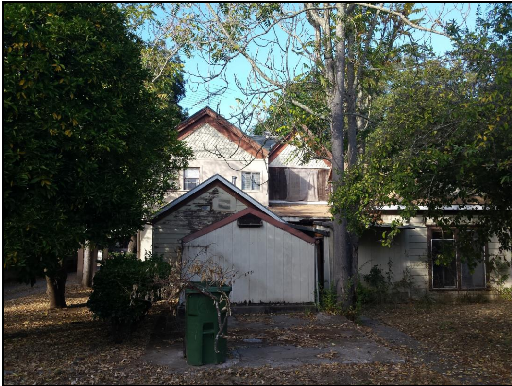
S (rear) elevation with multiple poorly-constructed additions, photo view toward N, 12/2017
