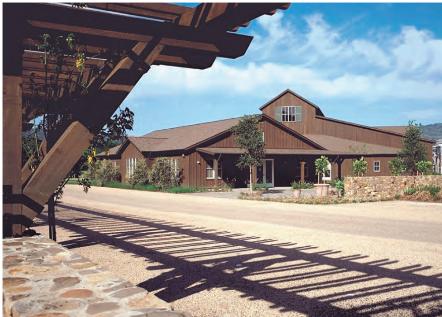
Vertical board and batten siding.
