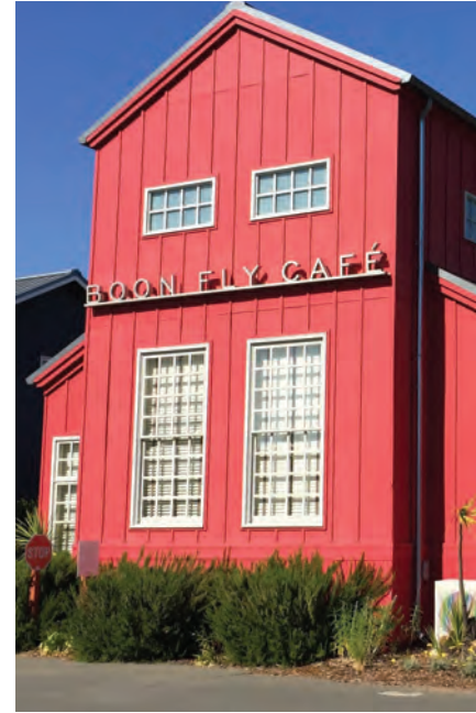
Multiple roof planes and divided windows add interest.
