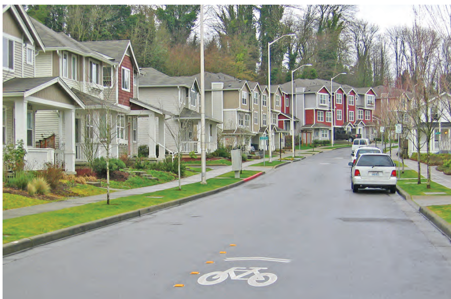
A road shared by bicyclists and vehicles, marked by sharrows.
