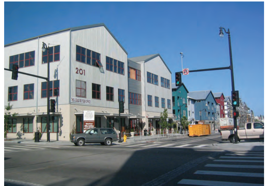
Corrugated metal siding.
